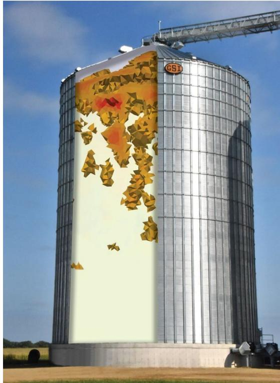
With the addition of the Winnipeg team, AGCO is developing GSI GrainViz using technology similar to an MRI scan to show the moisture content of grain inside a steel storage bin.
